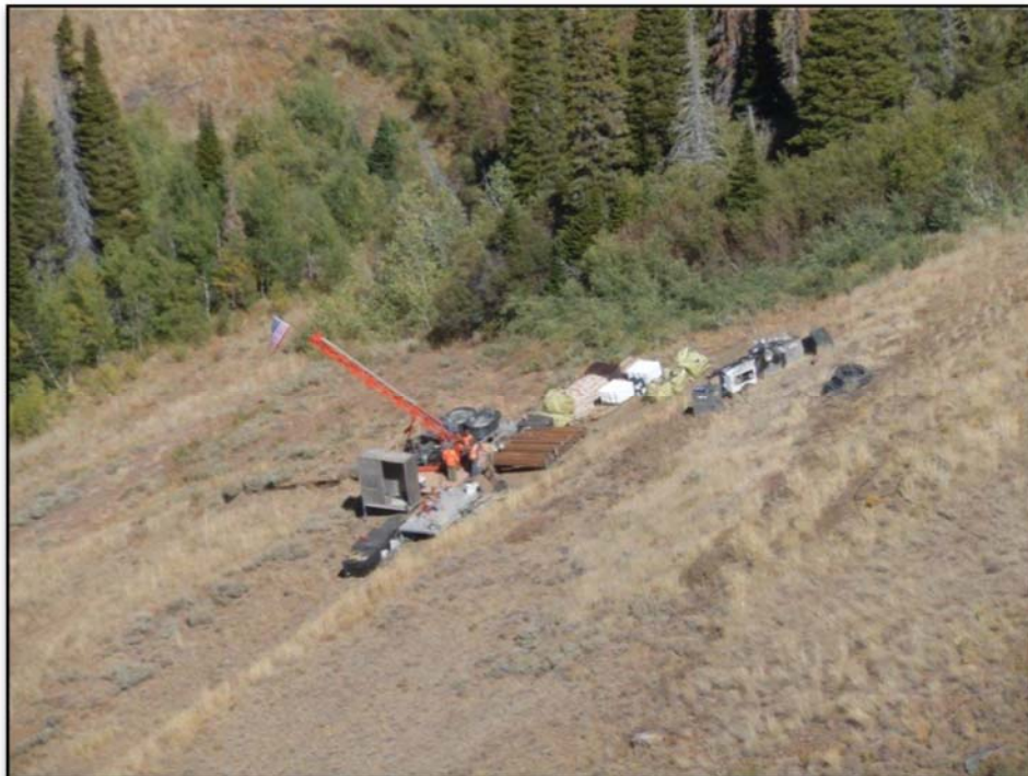
Image 1: Aerial view of drill rig at Beadles Creek
